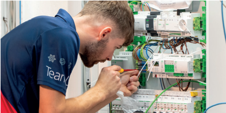
Electrical Installation competitor Jonathan Gough in action at the EuroSkills Herning competition in Denmark.
